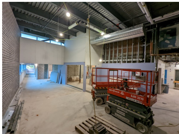
Interior: View towards the lower lobby area and accessible/family change room
